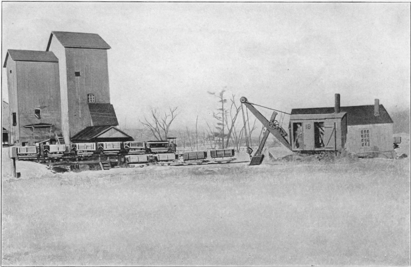
View of Crusher Buildings and Screen House showing Steam Shovel, Dump Cars, one of the Locomotives, and Shop
