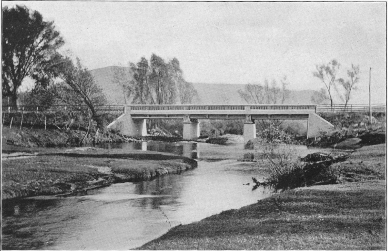
Concrete Bridge across Blackberry River at Canaan, Connecticut Slag furnished by the New England Slag Company
